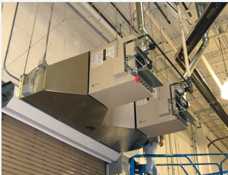
Indirect Gas Air Curtain | Custom Application
